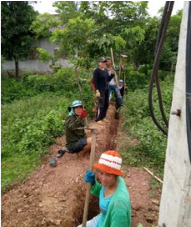
Community participation in water pipe laying in Namphone, Myanmar. Photo credit: Save the Children
