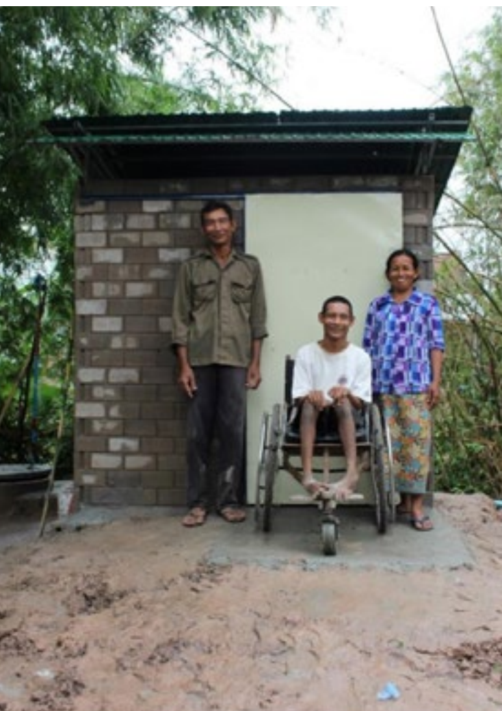
Interlocking brick toilet design for disability access latrine superstructure. Photo credit: iDE Cambodia
